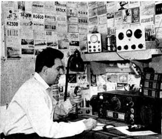
YO3GK is the only s.s.b. station active in Rumania. His equipment includes a transmitter running 40 watts to an 807, a 33 ft. Windom aerial and a 12 valve receiver.
